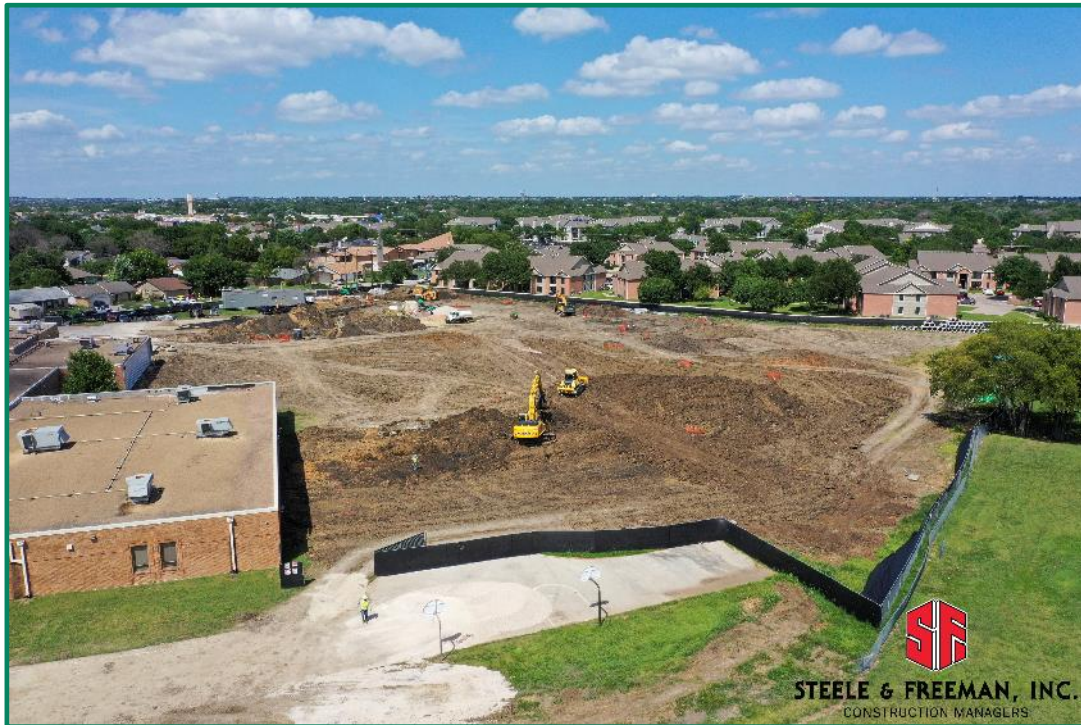
Site grading & temporary Fire Wall
