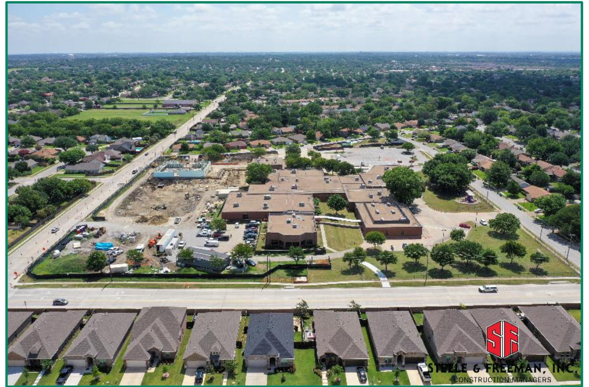
Temporary Bus Striping and sidewalk
