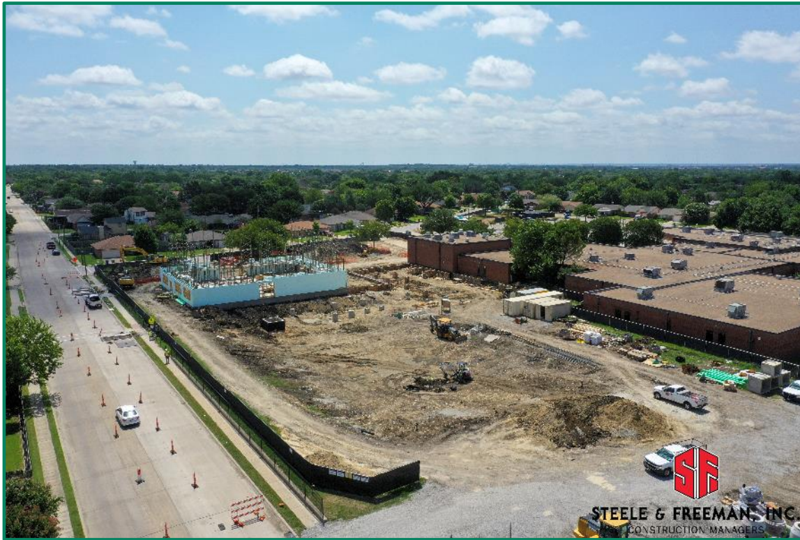
Storm Shelter Progress
