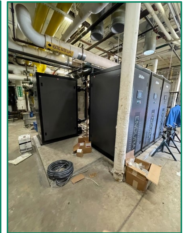
Hydronic Boiler Replacement for KHS
