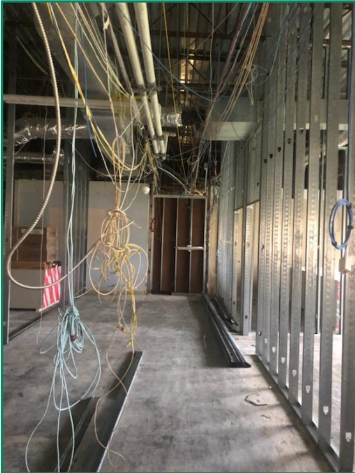
KCA construction progress
