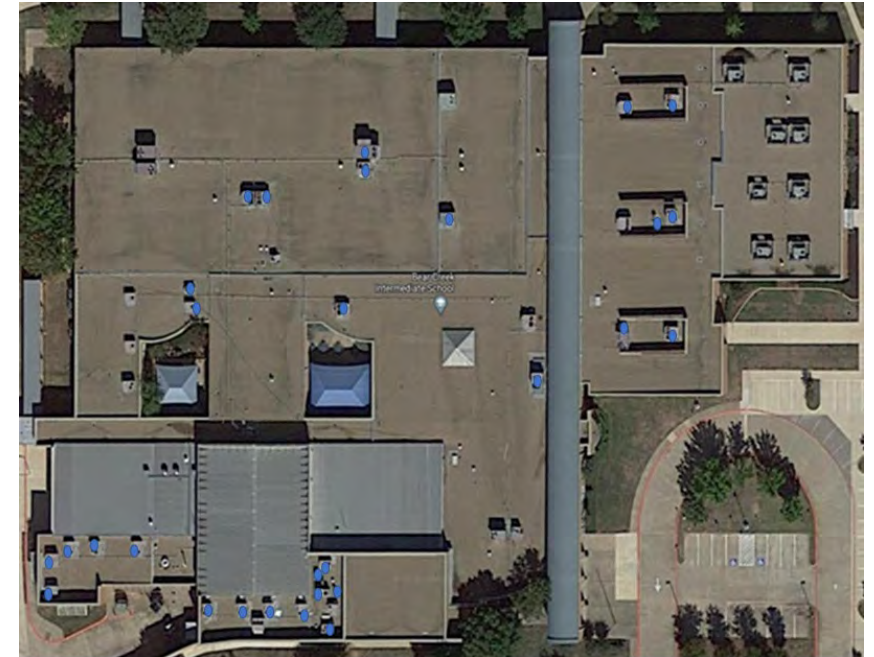
Bear Creek Intermediate Rooftop Unit Replacement
