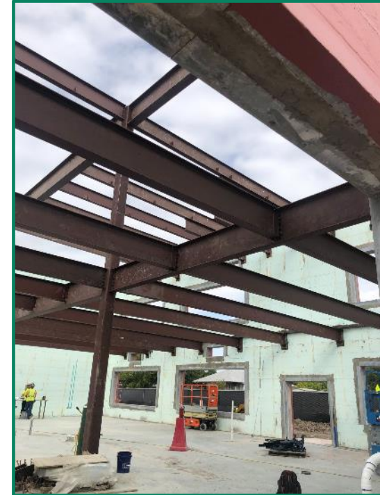
Storm Shelter Progress
