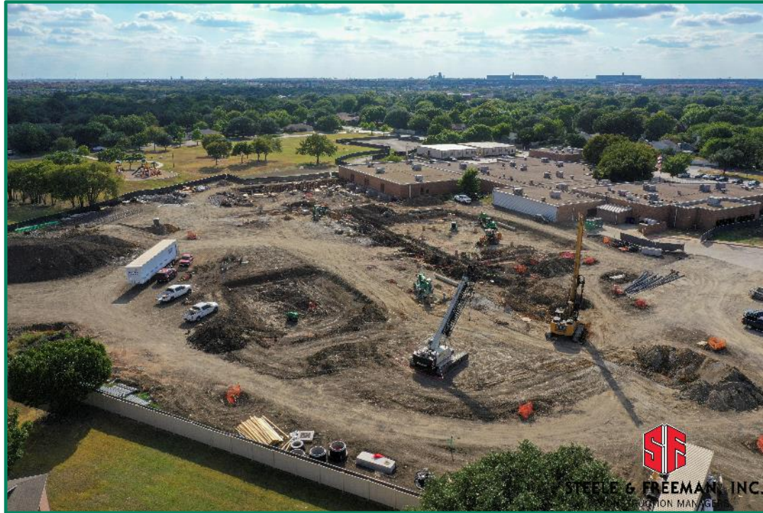
Piers and Foundation Progress
