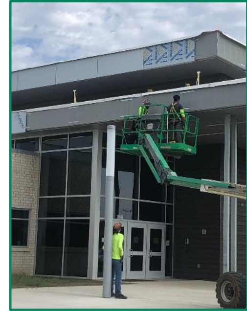
Aluminum Composite Material (ACM) Panel Install
