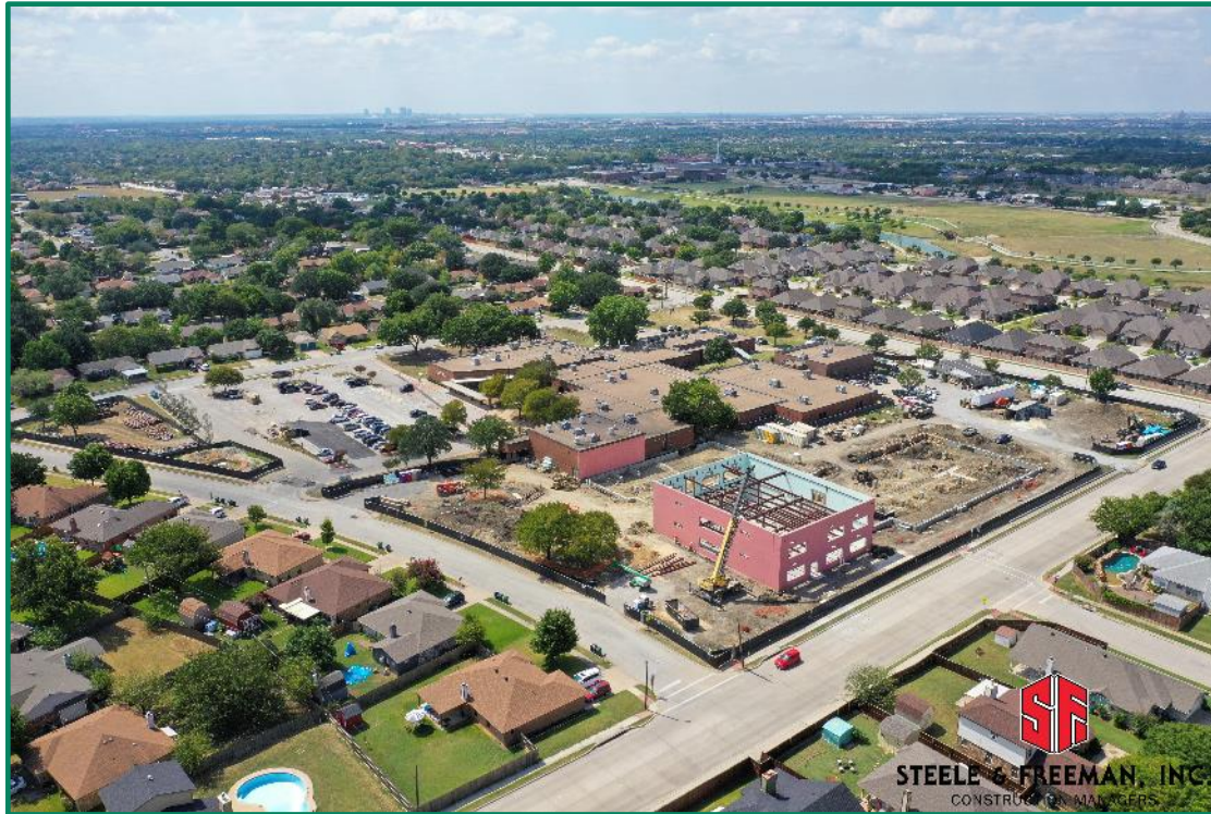
Storm Shelter, grade beams in progress
