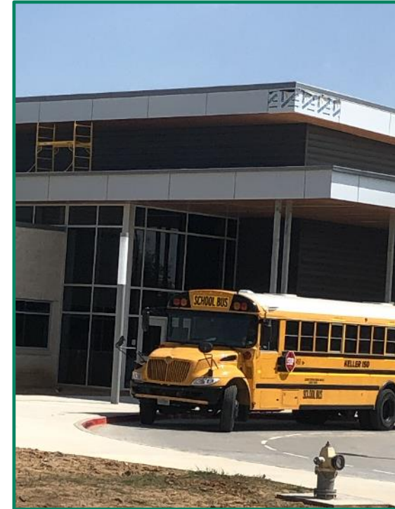
Aluminum Composite Material (ACM) Panel Install
