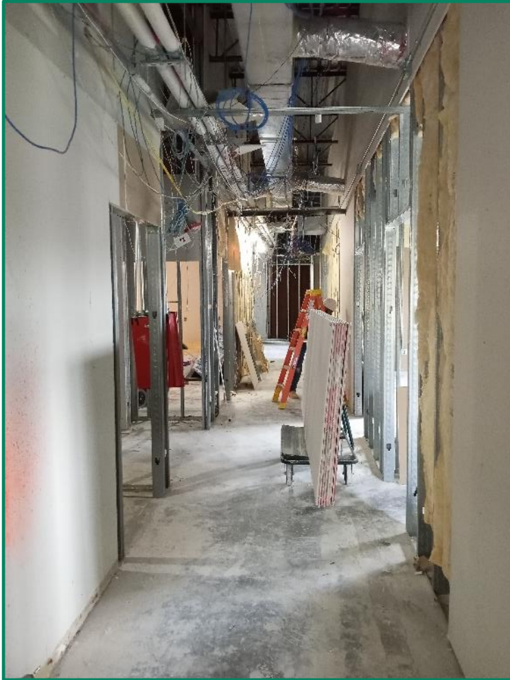
KCA construction progress
