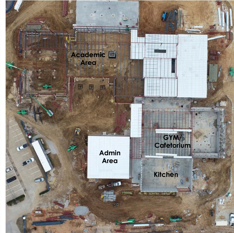
Admin roof and second floor decking
