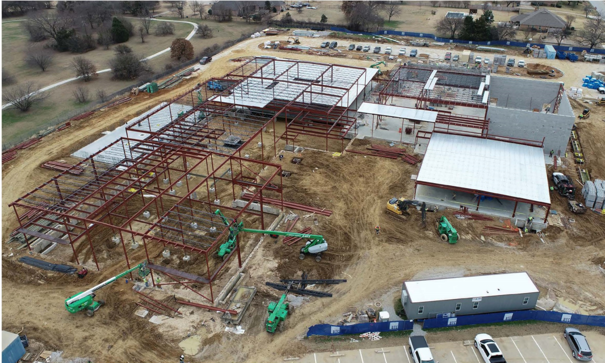
Progression of academic wing steel erection
