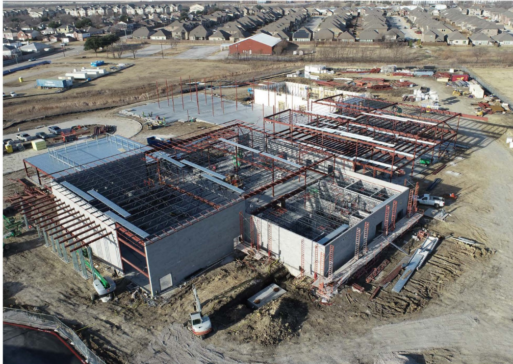
Masonry of gymnasium and kitchen
